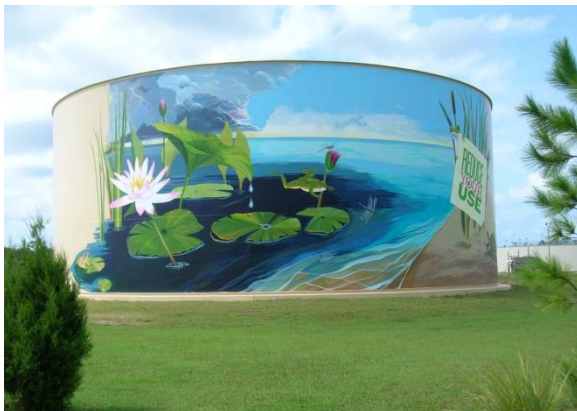
Reclaimed water storage tank completed as part of a project in the Southern Planning Region
