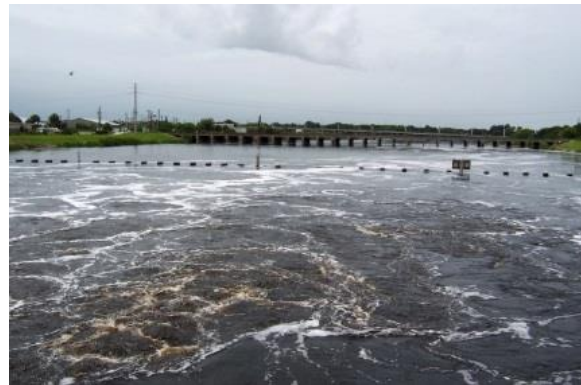
Tampa Bypass Canal
