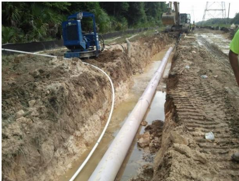
Construction of Crystal River to Duke Energy reclaimed water pipeline
