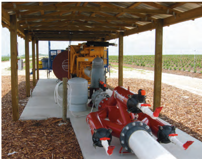
The FARMS Program is a partnership with state and federal agencies that provides cost-share funding for growers to install water-saving technologies. The District classifies FARMS as water resource development.
