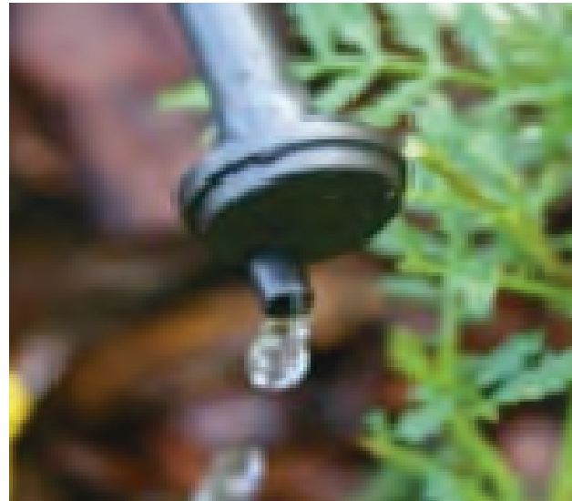
Use of a drip system to irrigate residential landscaping can help to reduce outdoor water use.
