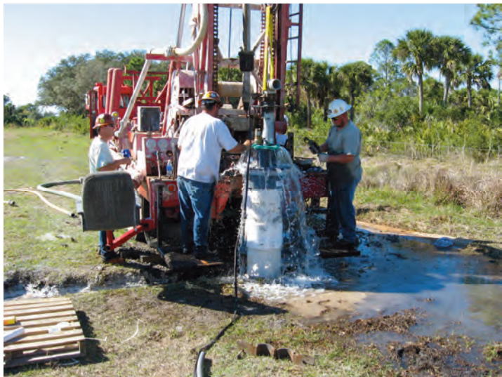
Construction of a groundwater production well.
