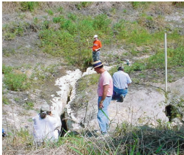
The karst berms project will evaluate the feasibility of constructing in-channel devices that will prevent dry-season river flow from being captured by karst features but will allow recharge to occur through the features during higher-flow periods.
