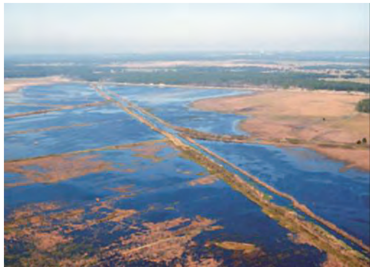
During 2004, several hurricanes that passed through the District caused severe flooding along Peace Creek in the headwaters of the Peace River.
