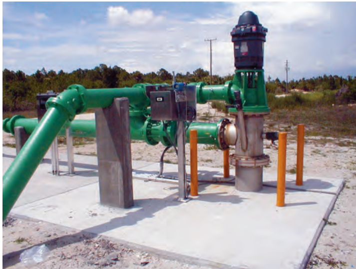
A typical aquifer storage and recovery well.
