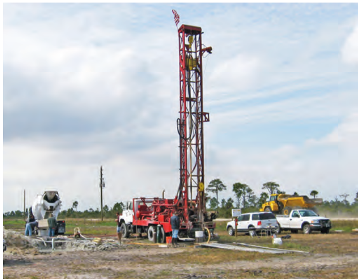
A large drill rig constructing a well into the Upper Floridan aquifer for agricultural irrigation.
