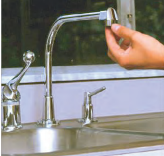
Easily installed faucet aerators are one of many ways to reduce residential water use.
