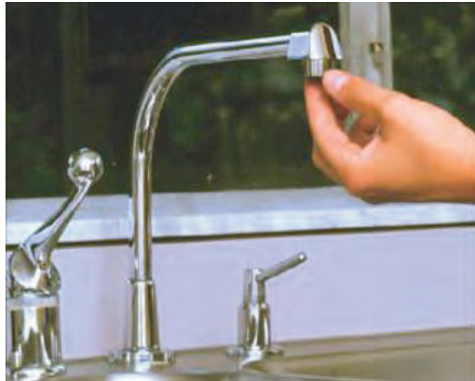
Easily installed faucet aerators are one of many ways to reduce indoor residential water use.
