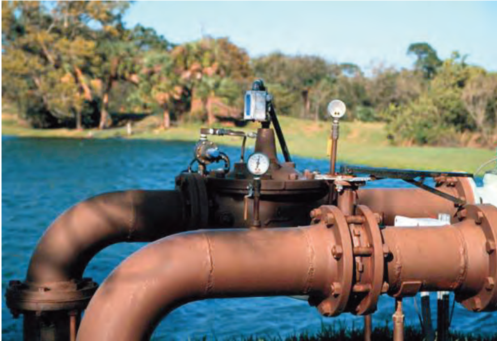
Reclaimed water is often pumped from the treatment plant into ponds on golf courses where it is used to irrigate fairways and greens.
