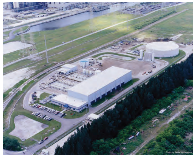
Tampa Bay Water's facility on Tampa Bay is the largest desalination facility currently in operation in North America.
