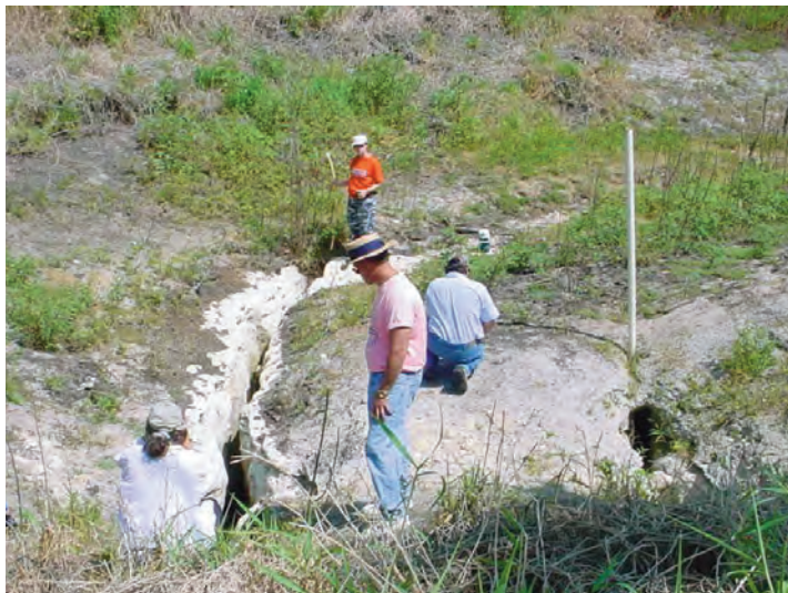
The karst berms project will evaluate the feasibility of constructing in-channel devices that will prevent dry season river flow from being captured by karst features but will allow recharge to occur through the features during higher-flow periods.
