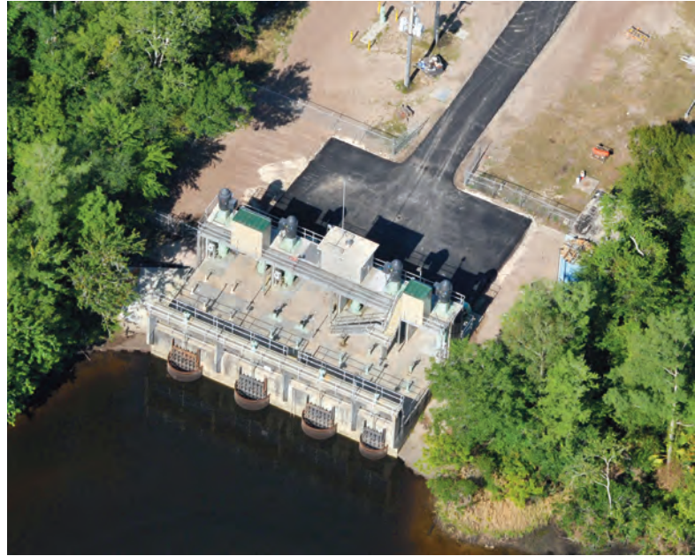
Aerial view of the Peace River Manasota Regional Water Supply Authority's recently expanded Peace River intake.
