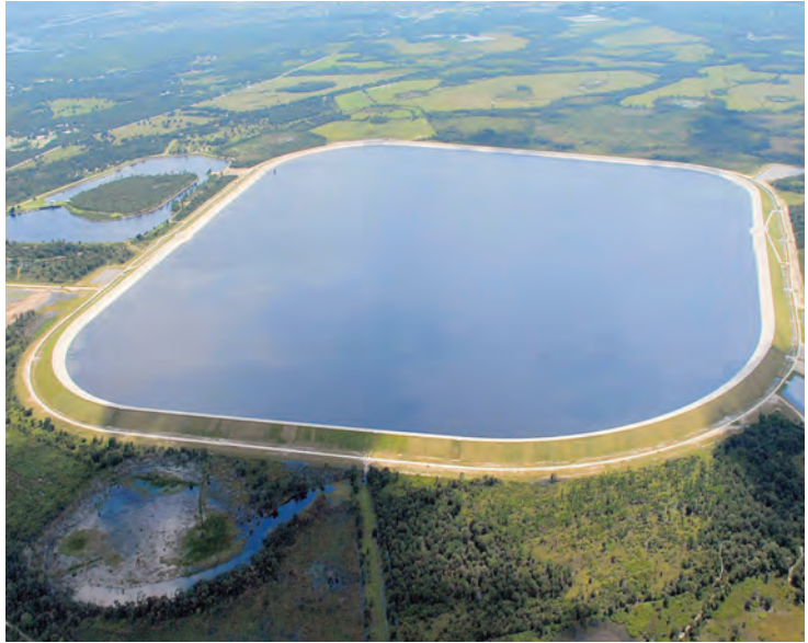
The Peace River Manasota Regional Water Supply Authority's recently completed 6-billion-gallon off-stream reservoir.
