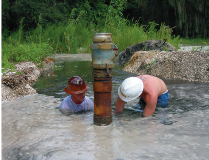
District technicians work to plug an abandoned free-flowing well.
