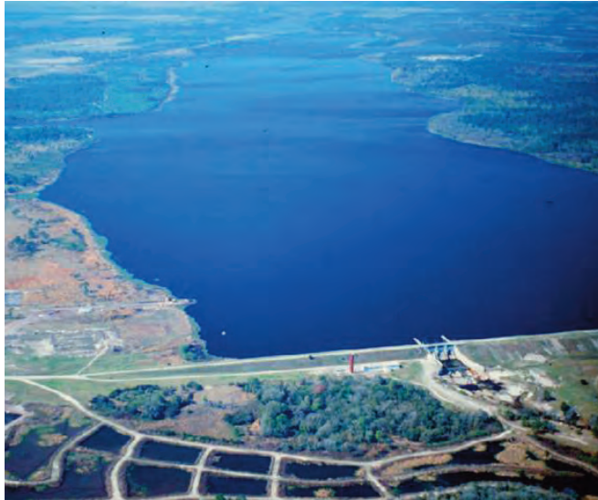
The dam on the Manatee River has created a reservoir that is a major water-supply source for Manatee County.
