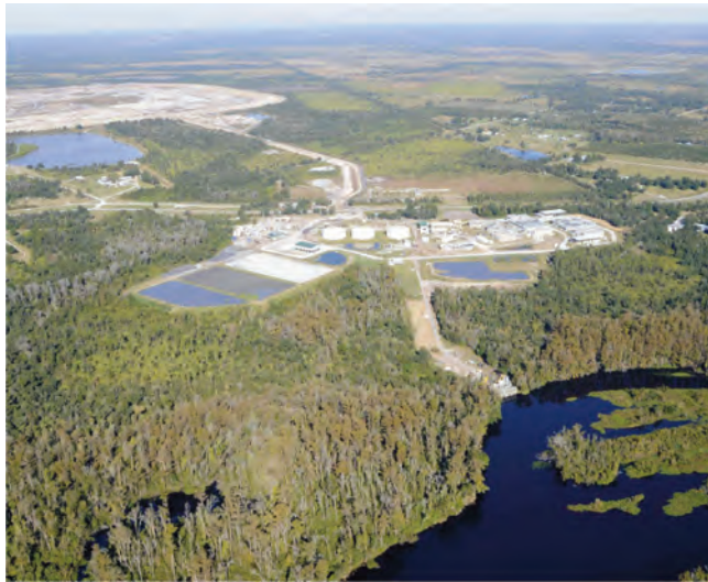
Aerial view of the Peace River Manasota Regional Water Supply Authority's Peace River facility showing the river intake, treatment facility and the 6-billion-gallon reservoir under construction in the background.
