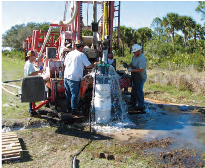
Construction of a groundwater production well.
