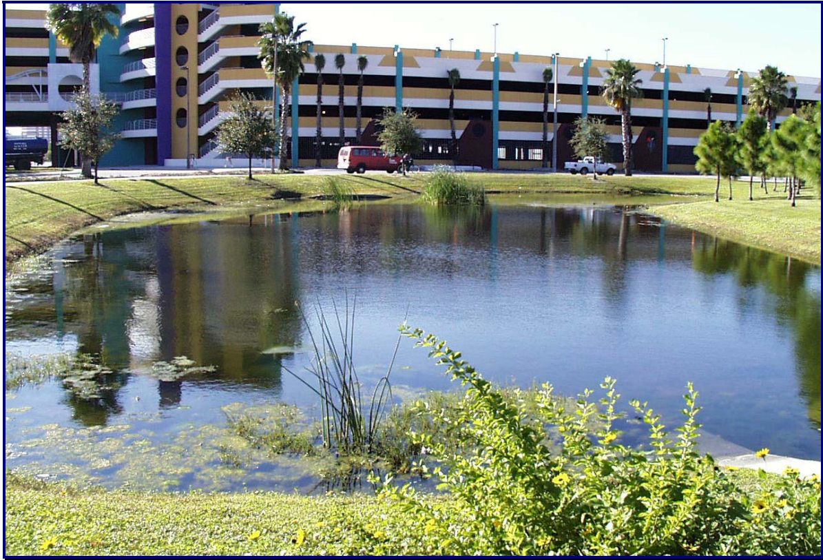
Picture 1 – Inflow (west view of pond) during Year 1 with new parking garage in background and before the littoral zone was planted.
