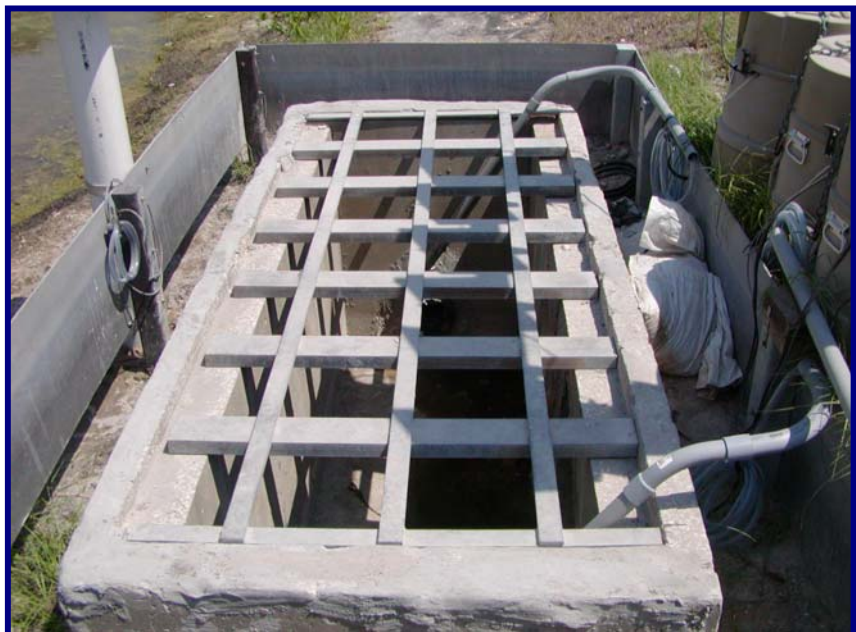
Picture 6 – Outflow weir and underdrains.
